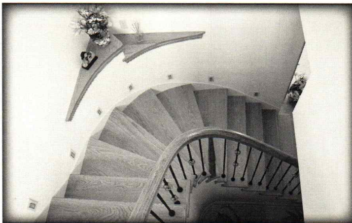
David steamed and bent the wood for their stair rail.
