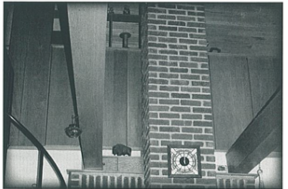
Beams encased with white oak harvested from one tree.
