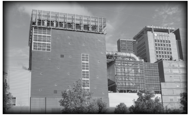
St. Paul District Energy located on the edge of downtown.
