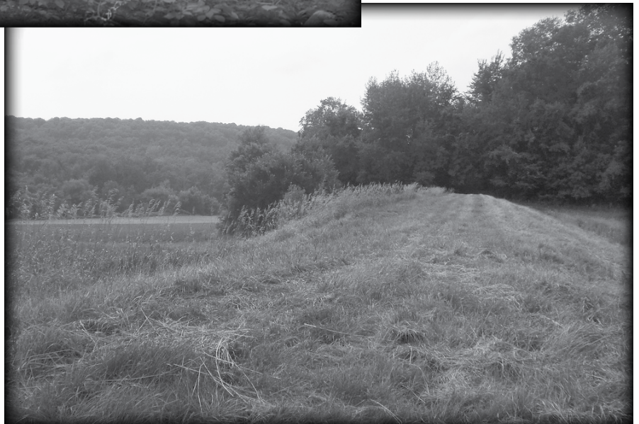
Below: An earthen dam on the Edlund farm helps manage runoff.
